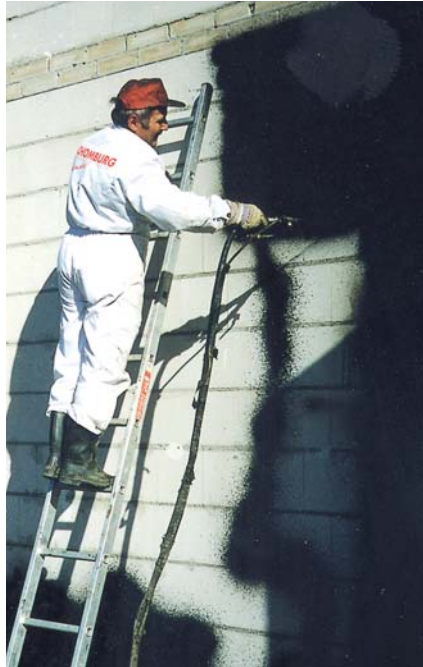
Waterproofing of a cellar wall with COMBIFLEX®-C2
