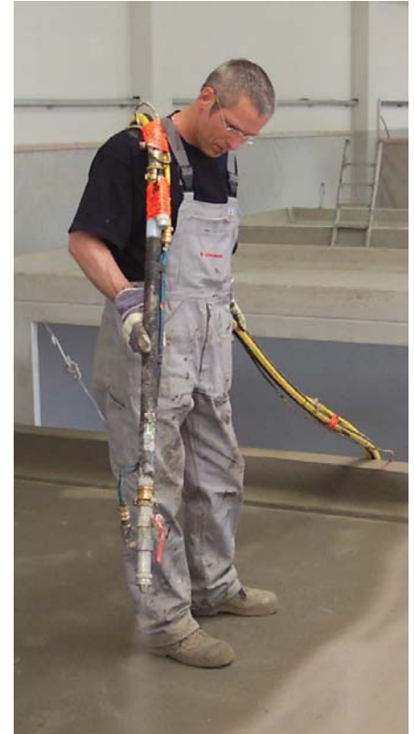
Waterproofing of a garage roof with AQUAFIN®-2K
